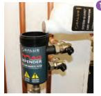
After step 9 in servicing, pour a bottle of water treatment corrosion and scale inhibitor, we suggest SALUS SYSTEM GUARD Inhibitor. The canister will hold 500ml and the inhibitor should be poured down the outer edge of the snorkel.
