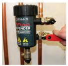
Important – Before carrying out any servicing work, turn off electrical supply to the boiler and let the water cool down to a safe working temperature. Using the Mag Defender spanner provided turn both isolation valves to the OFF position.
