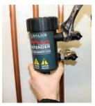
3 Loosely secure the Mag Defender to the valves. Grip the Mag Defender and tighten the compression fittings being careful not to over tighten as this may cause damage.
