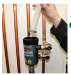
4 Withdraw the snorkel and mesh filter. Some debris may stick to the snorkel, however the majority will fall to the bottom of the canister.
