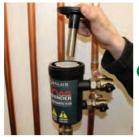
3 Remove the inner lid and magnet assembly.
