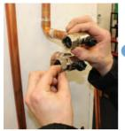
2 Now Loosen off the valve flange nuts and insert the rubber washers provided. (There are 2 supplied with this product).
